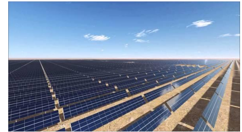
Pxhere Saudi Arabia PV farm
